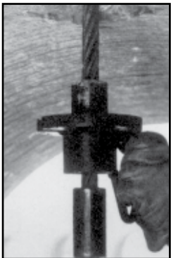
2. Align and insert "tea cup" pipe carrier into lifting sling.
